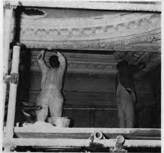
Working on the Drawing room ceiling
