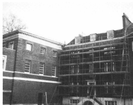
Renovation up College
