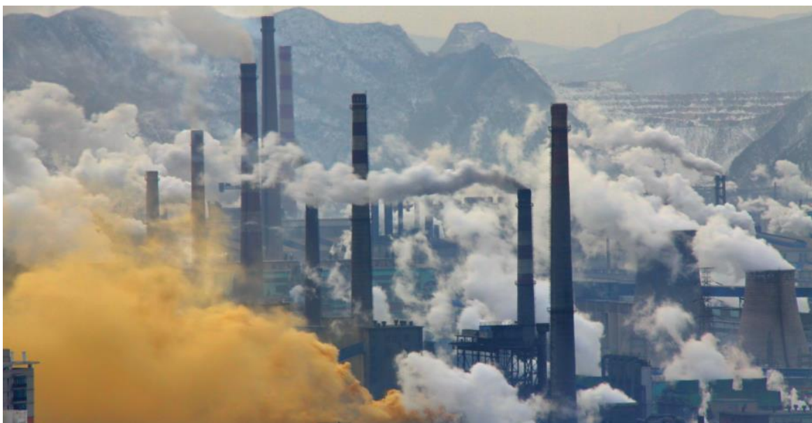
Benxi Steel Industries, Liaoning, People's Republic of China (Habich, 2013) https://chinaenv.colgate.edu/airpollution/air-pollution-in-china/
