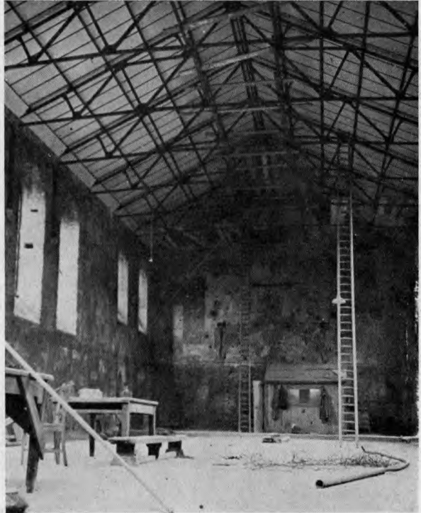
THE NEW ROOF
